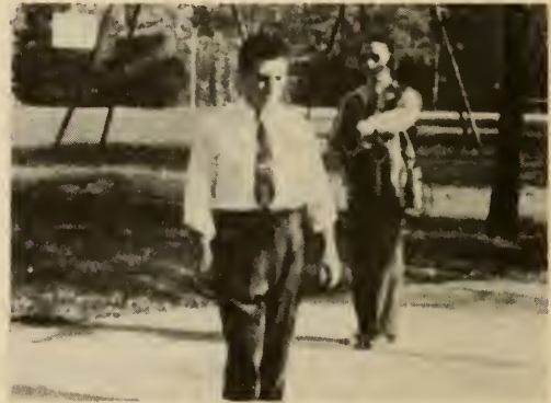
2-PEDESTRIAN CROSSING PATH, STROMBERG-CARLSON
